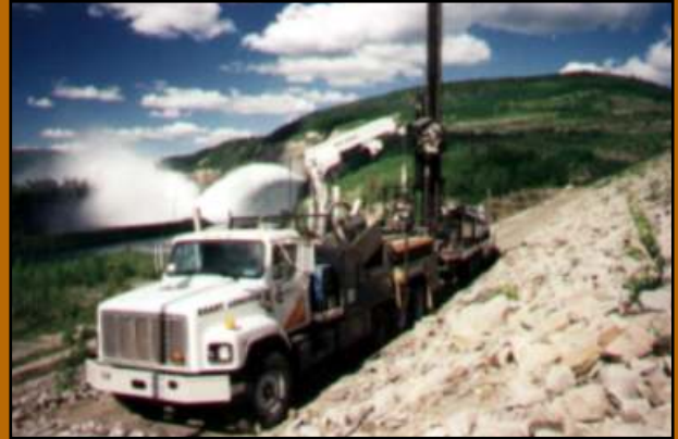
Sonic drill rig setup at the WAC Bennett Dam.
